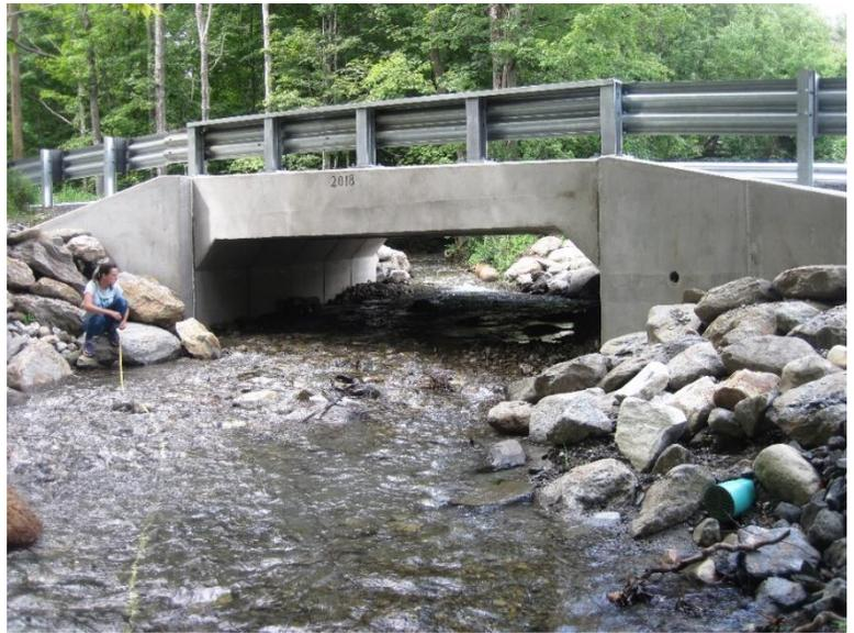
*Figure 2 Before (top) and after (bottom) photo of a culvert replacement project on Churchill Brook in Pittsfield, MA. The bottom structure is an-bottomed culvert that was designed with the natural stream channel in mind.*
