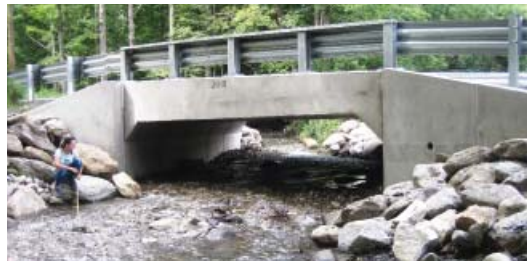
New culvert at Pittsfield's Churchill Brook
