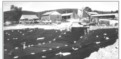
**Above: Workers lay down the impervious, heavy-duty liner in the manure pit below the barnyard and away from Sucker Brook to eliminate wastewater infiltration.**
