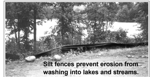
Silt fences prevent erosion from washing into lakes and streams.
